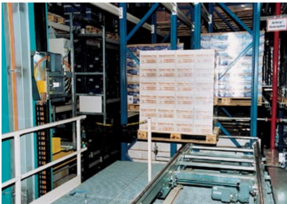
Automatic conveyor technique of the high rack warehouse
