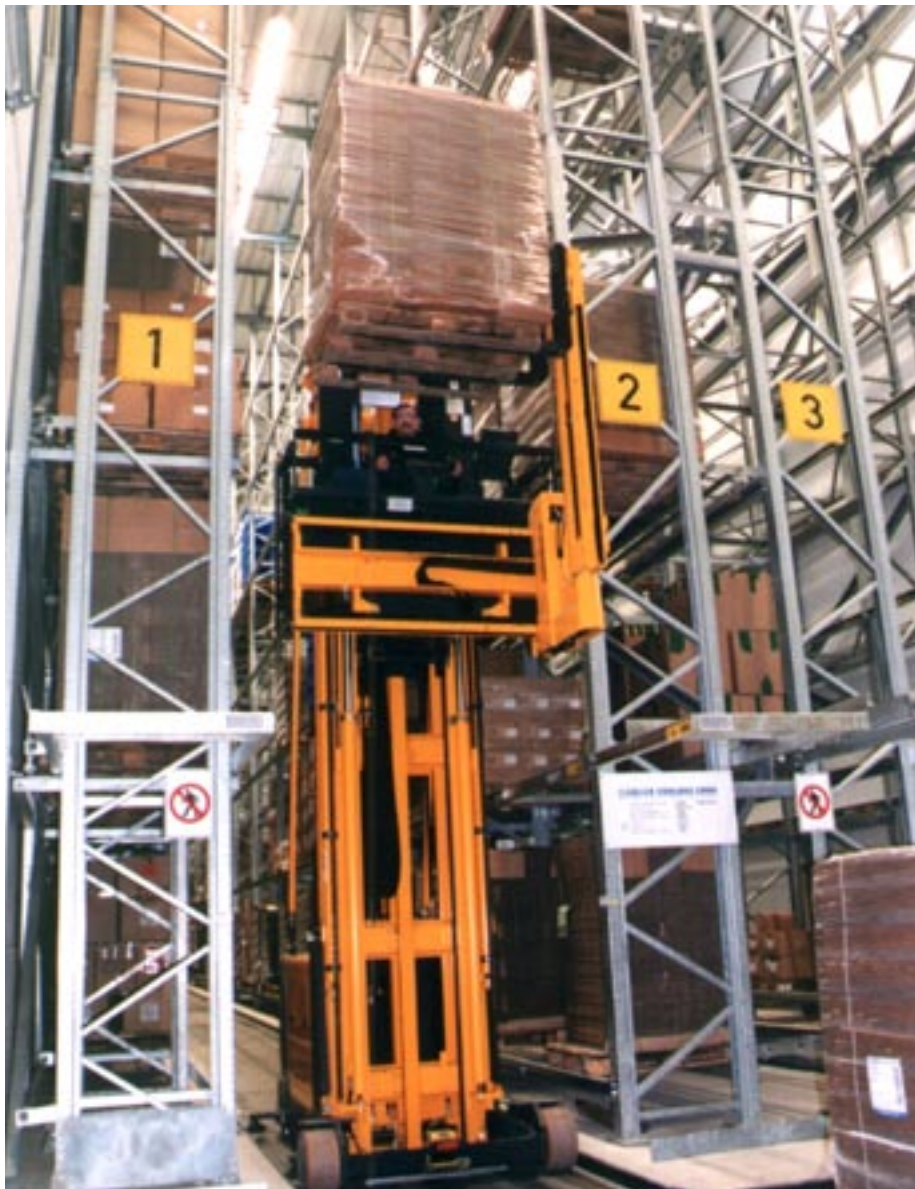
High-bay area in the stacker crane (rack head)
