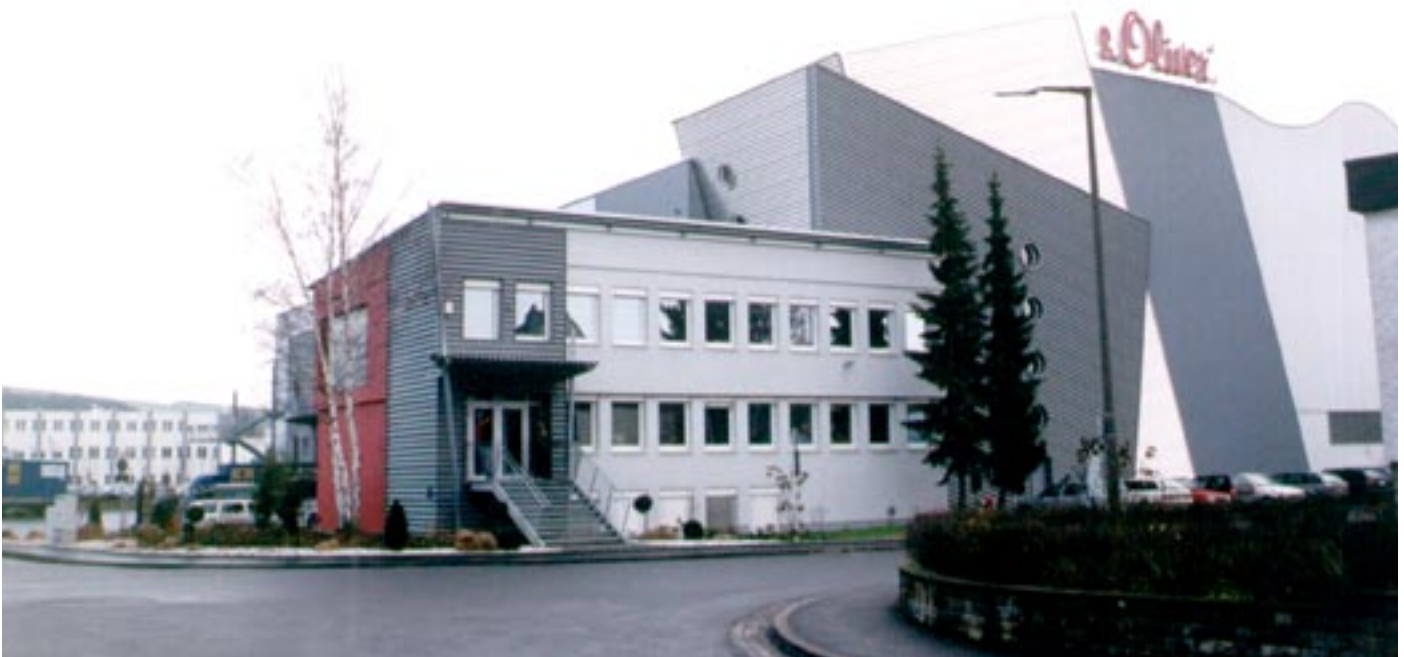
Logistics centre in Rottendorf near Würzburg/Germany
